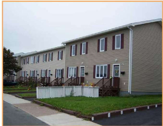
Salter Place modernization
